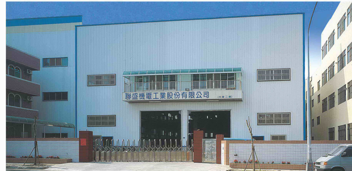
◆ THE NEW SECOND PLANT
